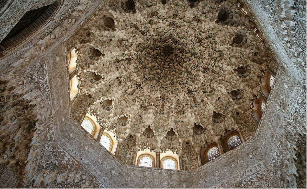
Muqarnas stalactite vault, Sala de las Dos Hermanas, Palace of the Lions, Alhambra, Granada, c.1380. Approximately 5,000 individual carved plaster cells arranged across 16 radiating arms, transitioning the square plan of the hall into a circular, skylit crown. The poet Ibn Zamrak's verses, inscribed in the frieze below, describe the vault as the heavens in motion.
