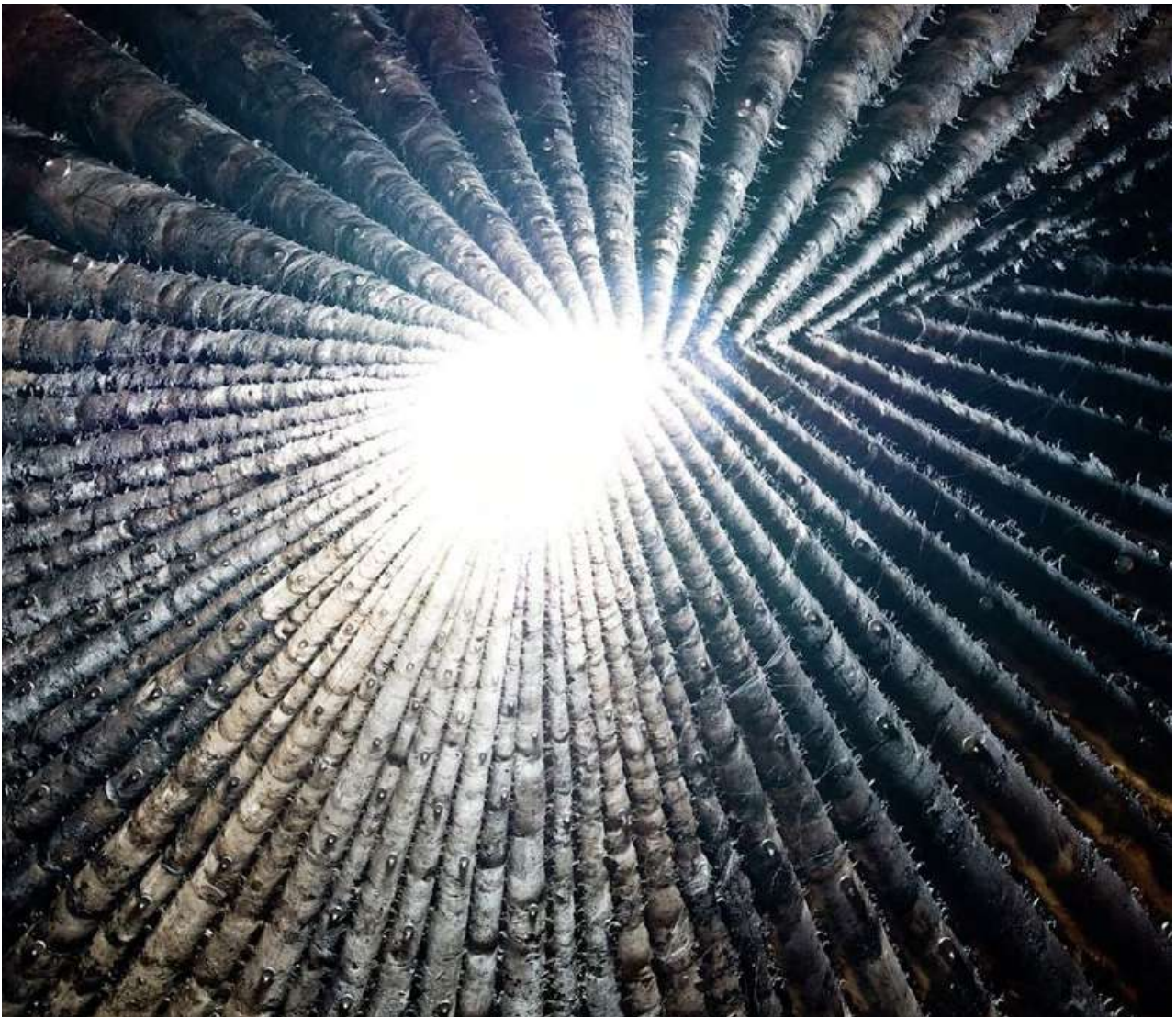
Bruder Klaus Field Chapel, Peter Zumthor, Wachendorf, Eifel, Germany, 2007. Interior looking toward the oculus. The cavity was formed by burning 112 tree trunks from within the completed concrete shell over three weeks. Floor: cast lead. Photography by © Samuel Ludwig via google.
